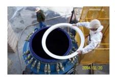
The glass lined vessel failed twice after 14 months of service operating at 145 degC and -0.5 bar g pressure due to because the corrosion of the 37%-42% sulfuric acid.
