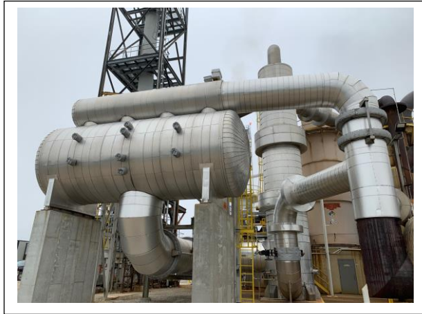
Figure 1. Heat exchanger in the cold position
